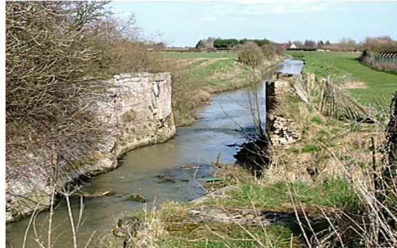
Salterfen Lock - approach from upstream
