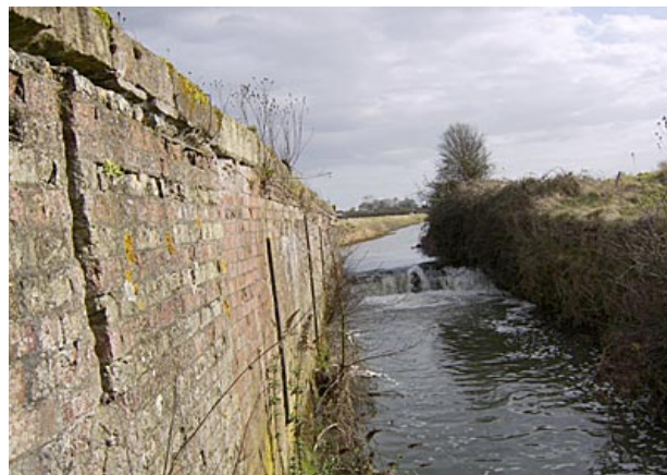
Outfen Lock - South Wall with Cill
